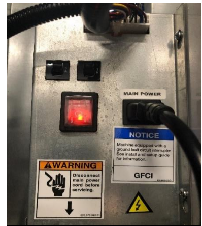
AC Distribution Box
